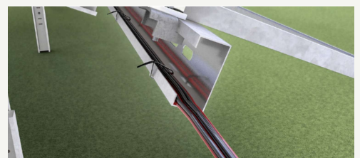
10. Cable management holes in purlins for easy and efficient cable securing
